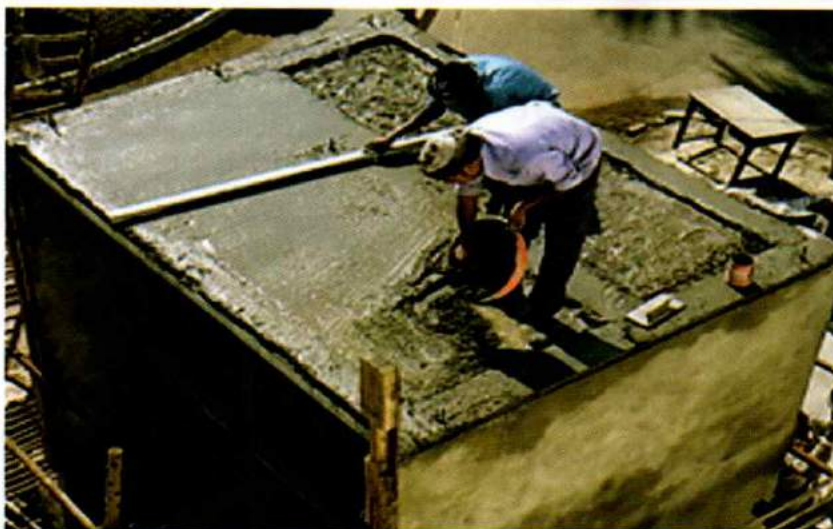
Spraying and pouring of concrete over the EPS core skeleton and finished building model
