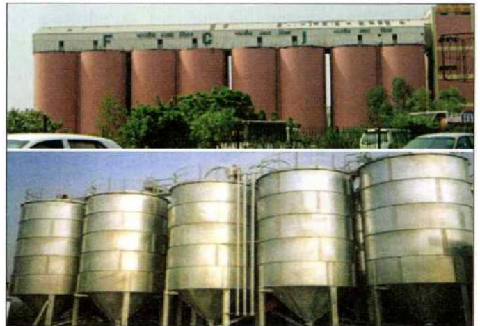
Fig. 3: Concrete silos at FCI, Mayapuri, New Delhi, and Commercial hopper bottom storage silos
